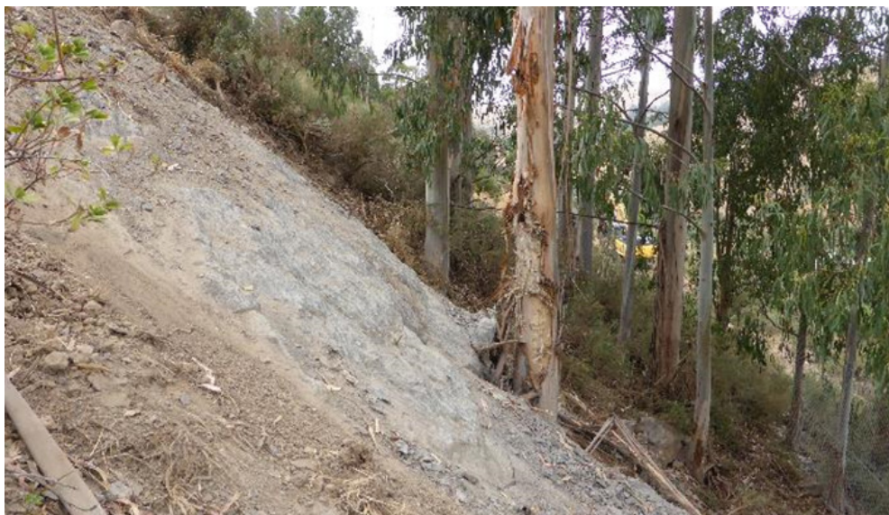
Figure 3. Case study 2: Example of rock source milled back to slope, Bowenvale Valley.
