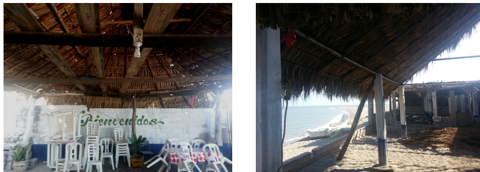
Figure 2. Left: Interior of a timber-roofed building with randomly mixed RC and timber columns and a single unreinforced masonry wall. Right: improvised wooden posts against poorly connected RC columns of the same building (Photos by S. Ortiz-Palacio)
