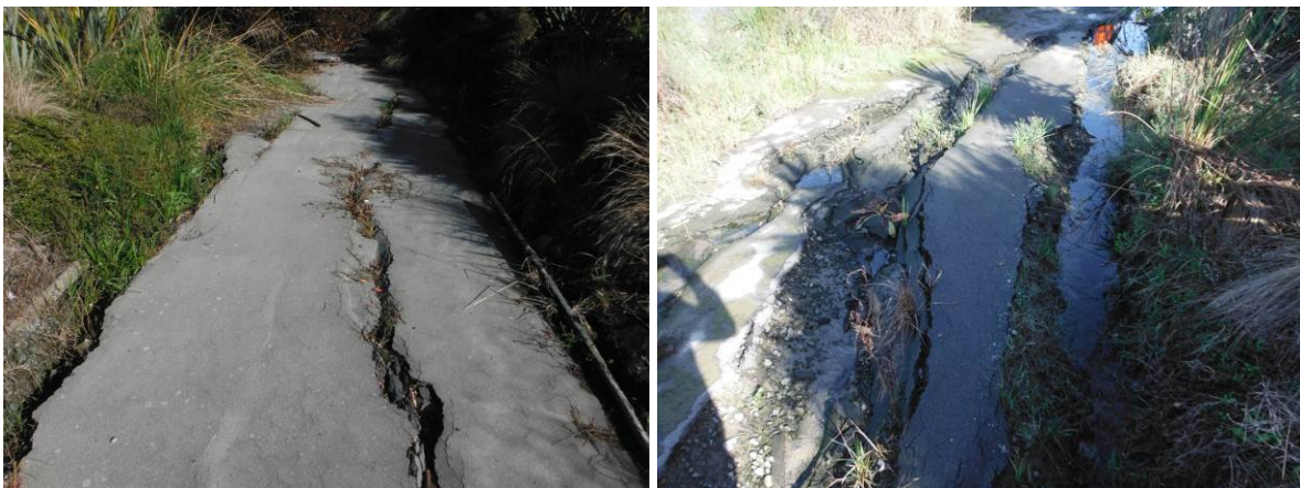
Figure 3 Footpath beside north abutment
