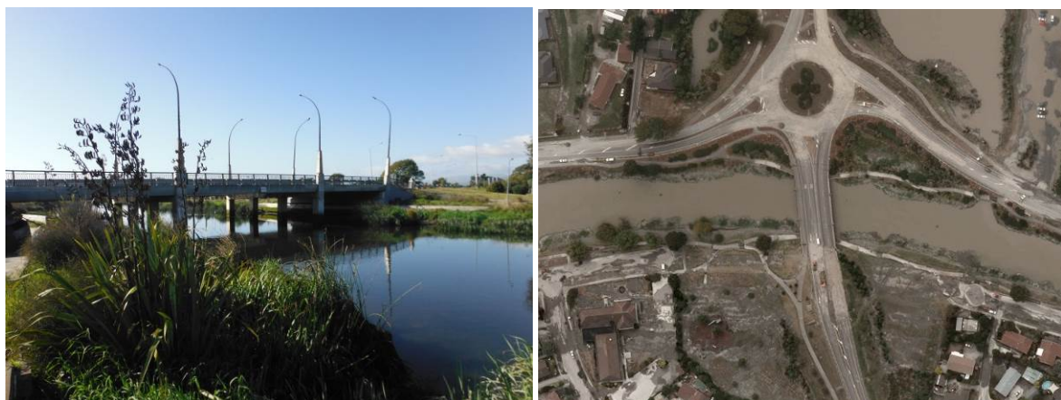
Figure 2 Anzac Bridge from bank (left) and aerial following Feb 2011 Earthquake (right)
