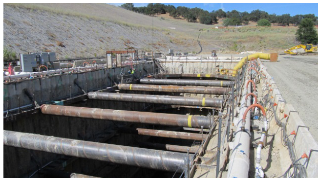
Figure 2. Key-block construction of single cell using structural wall system
