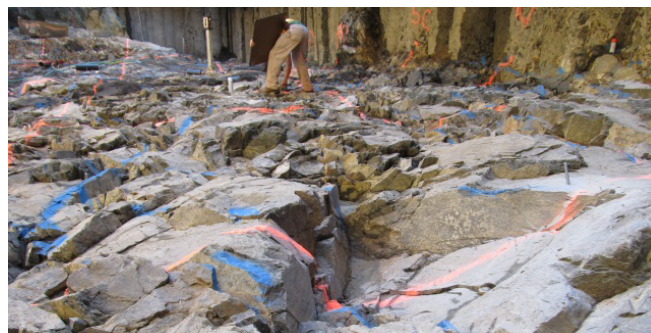
Figure 3. Key-block foundation excavated and cleaned bedrock surface being mapped
