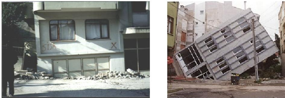
Figure 1. Liquefaction induced damage during the Kocaeli earthquake of 1999 in Turkey (adapted from Madabhushi and Haigh, 2009)
